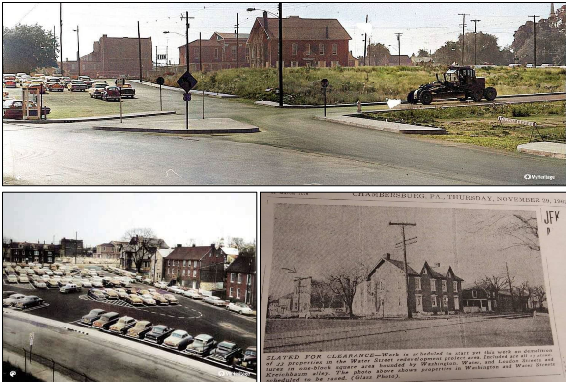
Figure 2-4: Water Street Redevelopment Project, Circa 1962
